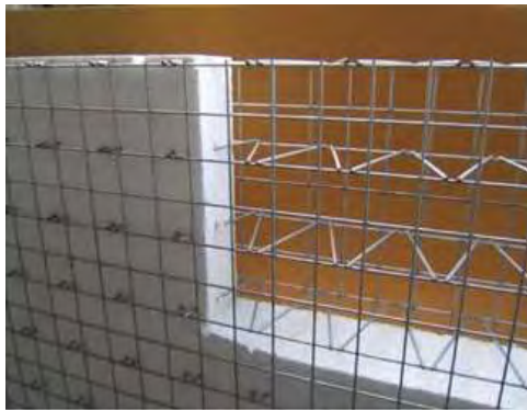
Fig 1.2: Reinforcing mesh expanded polystyrene core and diagonal wire.
